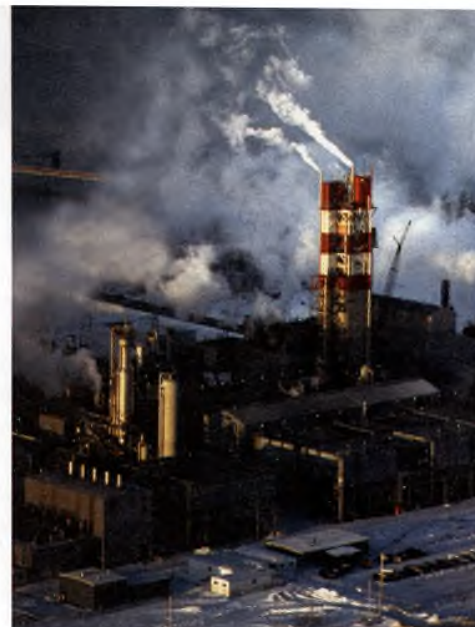
Figure 27 Operating an ammonia plant at relatively low temperature, high pressure, and low ammonia concentration maximizes the amount of ammonia produced.
