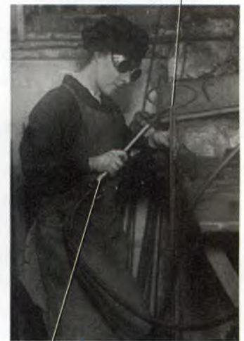
Gas torch GAS WELDING
