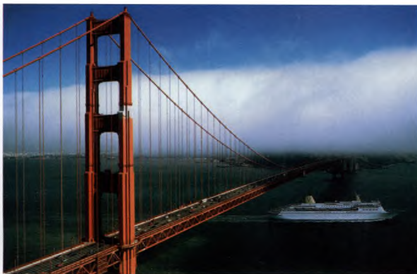
Figure 24 The Golden Gate Bridge is a landmark in San Francisco, California. Its cables, towers, and deck contain steel. The steel in the cables needs to resist forces that pull on the cables. The steel in the towers needs to resist the compression forces caused by the weight of the cables, the deck, and the vehicles that travel across the bridge.
