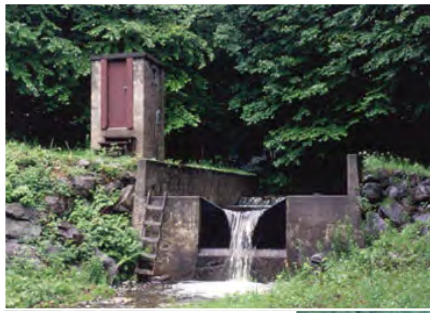
(a) Concrete dams and weirs built across streams at the bottom of watersheds enabled researchers to monitor the outflow of water and nutrients from the ecosystem.
